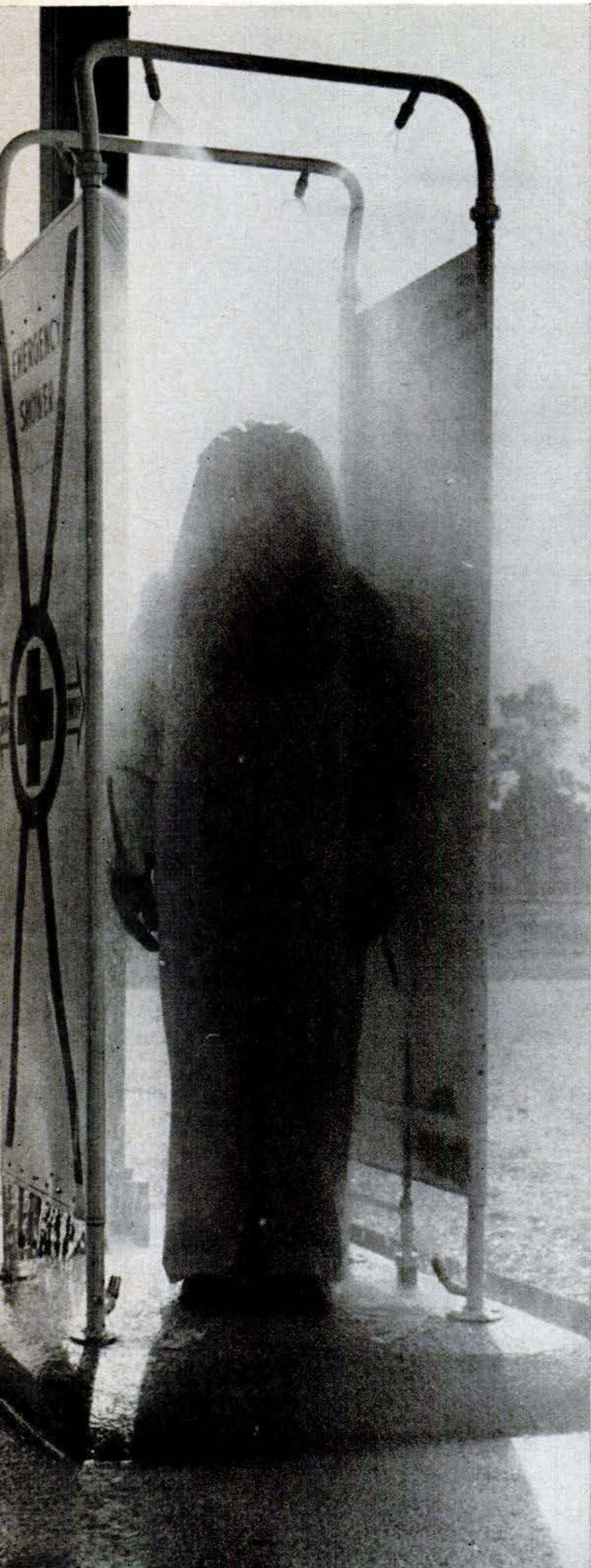
ACCIDENT INSURANCE THAT PAYS OFF FAST: Emergency showers are on tap close to crew that handles hazardous fuel for the Rascal missile.
